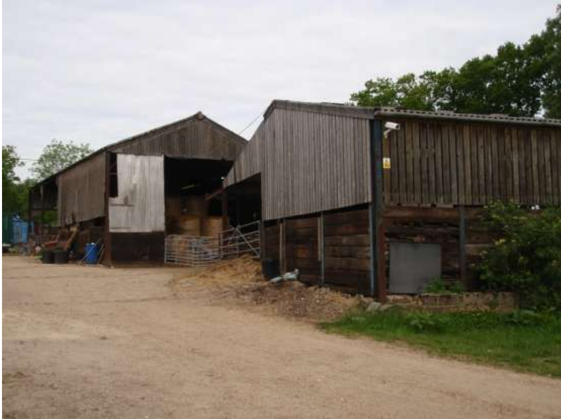
Plate 17. The farm (looking west)
